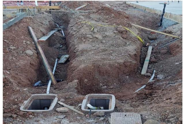
*Common incorrect practice of improper materials being left in a trench before backfilling*
