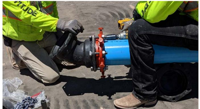
*Installation of proper fittings for a PVC water main connection*
